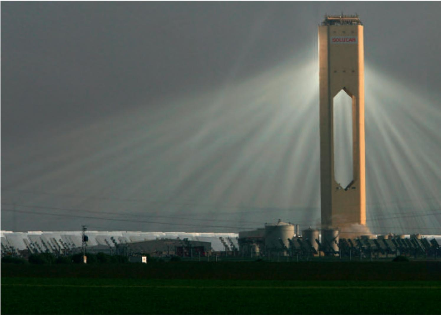
In southern Spain, Abengoa Solar's PS10 tower concentrates the light reflected from 624 mirrors. The world's first commercial solar tower generates 11 MW
